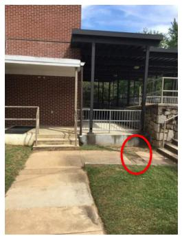
**Description:** Section of concrete walk needs to be repaired in courtyard
