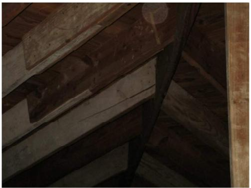
Photo 32: Cracked Roof Rafter at Northwest Corner of Northwest Classroom/Stairwell
