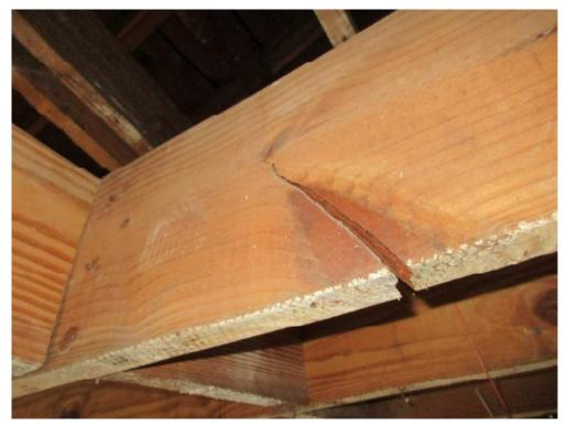
Photo 29: Typical Cracked Ceiling Joist
