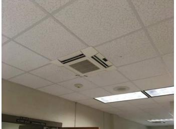
**Description:** Existing HVAC system is VRF with dedicated outdoor air units. Dedicated split system fan coil units are provided for IT/Data rooms. A new building automation system was also provided.
