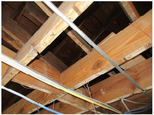
Photo 30: Typical Cracked Ceiling Joists
