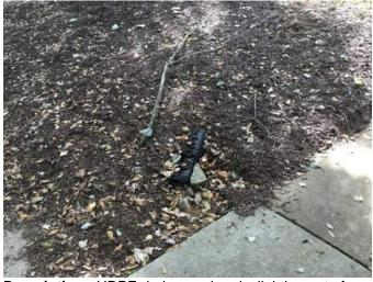
**Description:** HDPE drainage pipe daylighting out of grade destroyed
