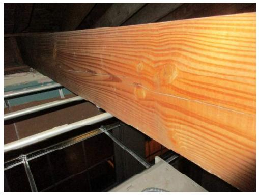
Photo 31: Typical Split Ceiling Joist
