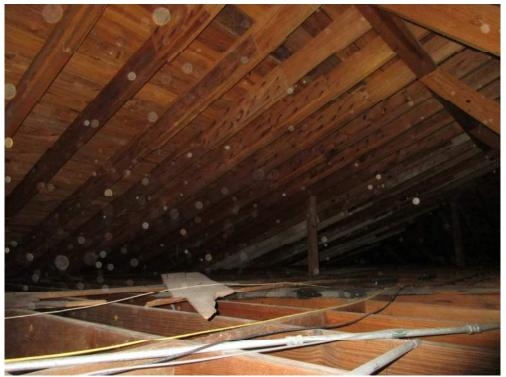
Photo 14: Typical Structurally Inadequate 1949 Roof Rafter Splice Locations at Midspan
