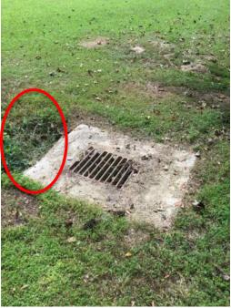
**Description:** Signs of soil failure around drop inlet in play field
