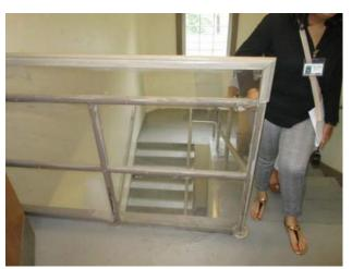
**Description:** Railings in existing typical exit stair do not meet current Life Safety codes.
