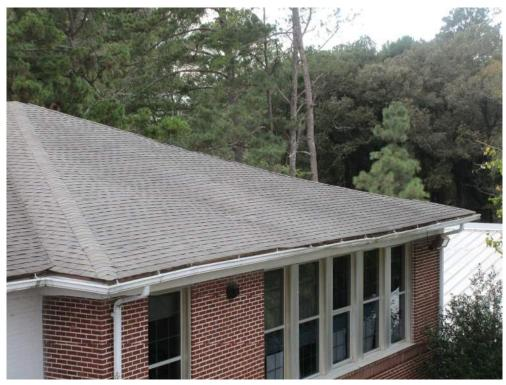
Photo 7: Visible "Sagging" of Northeast Classroom Roof
